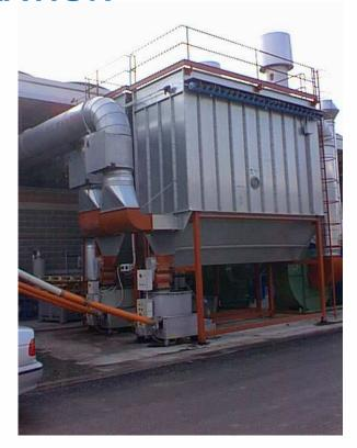
The whole dust suction system is connected to an external air system.
