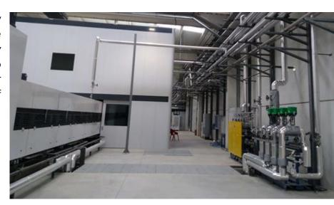
Digital steam pumps make free pressure regulation compatible with the simultaneous optimization of thermal transfer: in each single facer or hot plates section, its digital pump collects the condensate and pumps it with steam to its general recovery towards the boiler.
