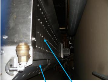
Water Spray System 4 Row of Nozzles Water Spray System
